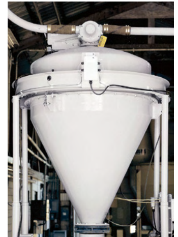
Scale hopper with Aeropass valve
